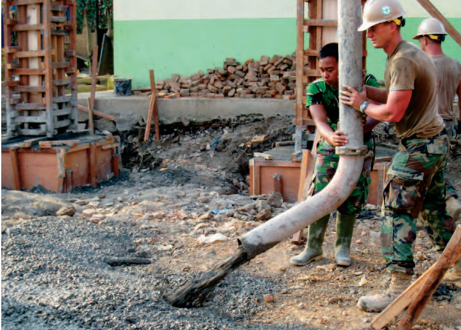
An Indonesian navy engineer and a U.S. Navy Seabee from Naval Mobile Construction Battalion 40 pour concrete for an engineering civic action program during the first phase of Cooperation Afloat Readiness and Training Indonesia 2009. Warfighters get the construction materials, fuel and other sustainment supplies they need during regular and humanitarian operations from the Defense Logistics Agency-Pacific Region team.
